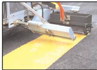
All steel extrusion dies up to 18" wide.
